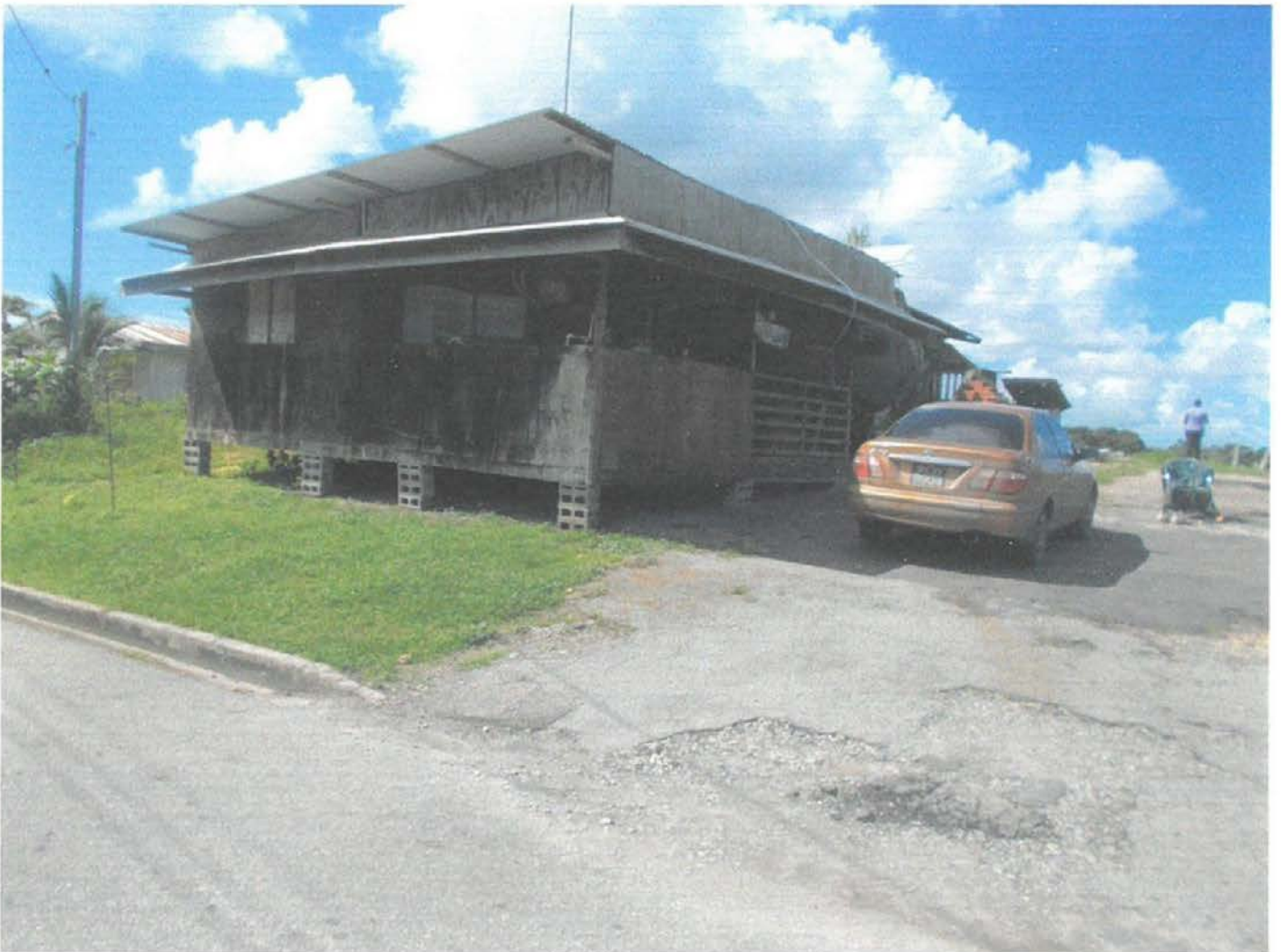
SITE VIEW OF ONE-STOREY
