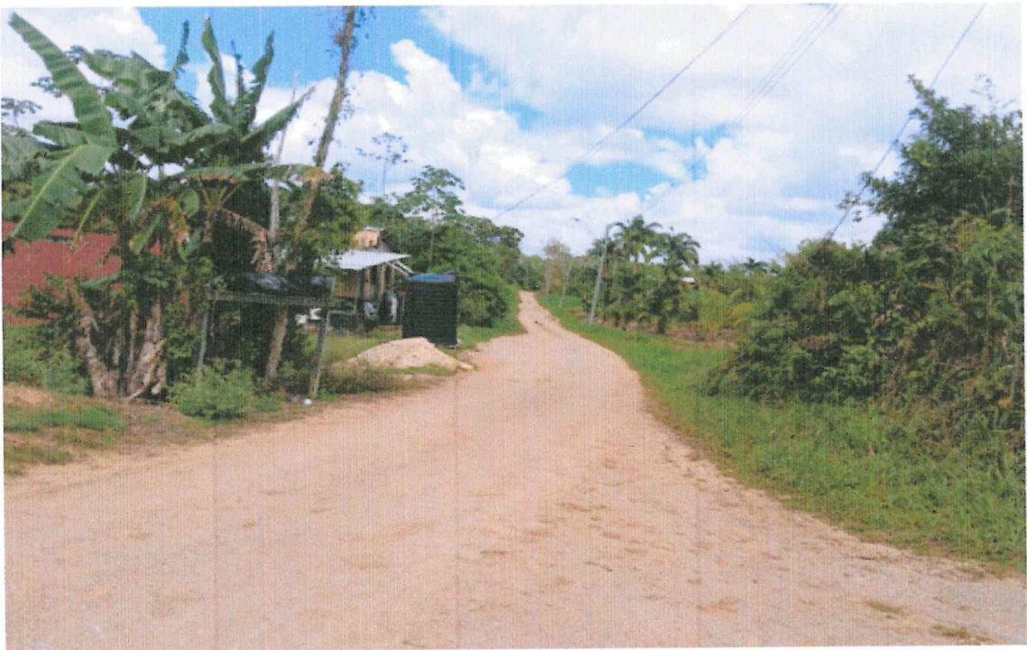
GLOD ROAD VIEW LOOKING EAST
