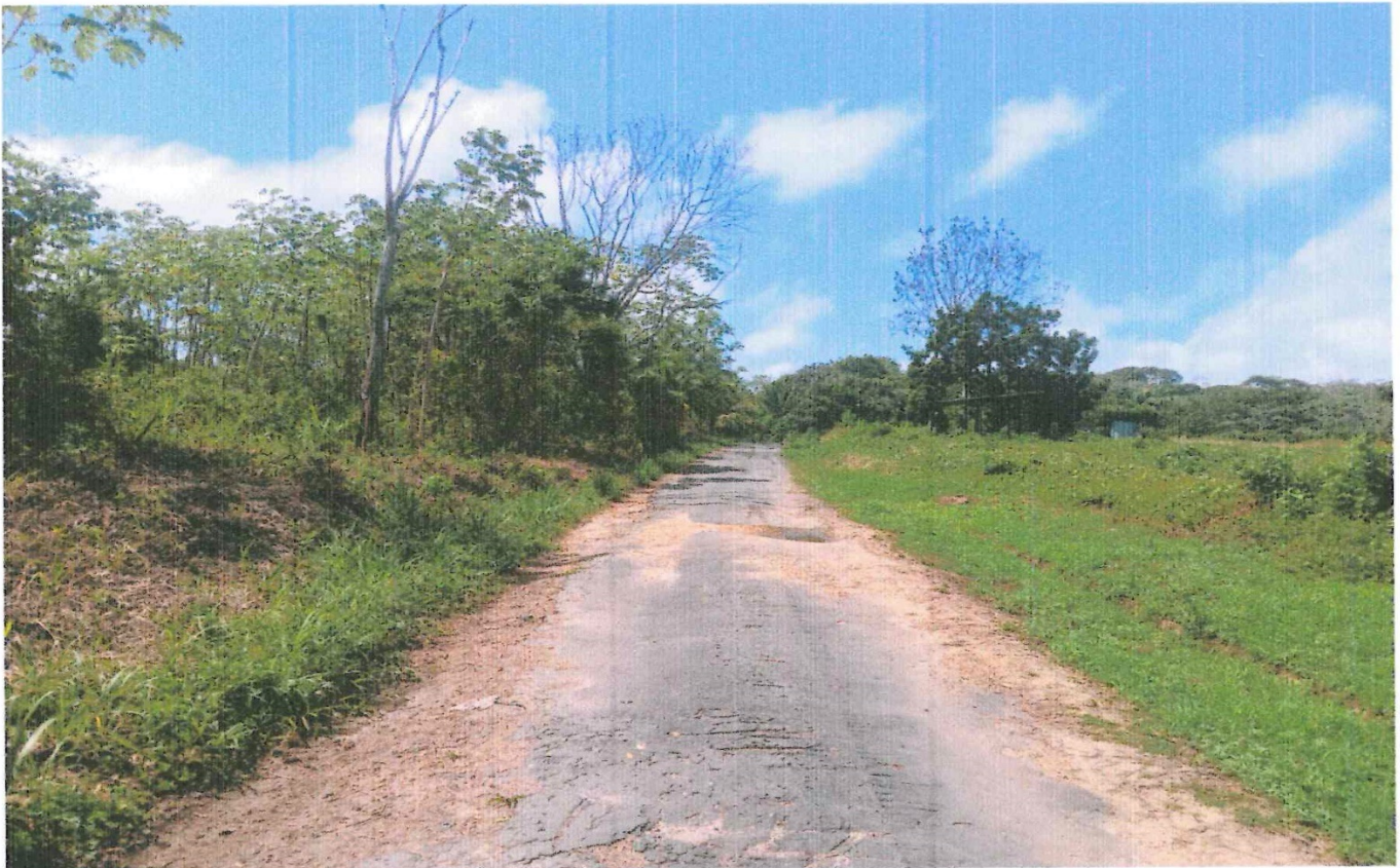
ROAD VIEWS LOOKING SOUTH
